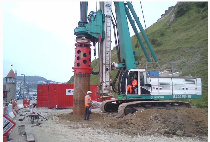
August - installing concrete columns
