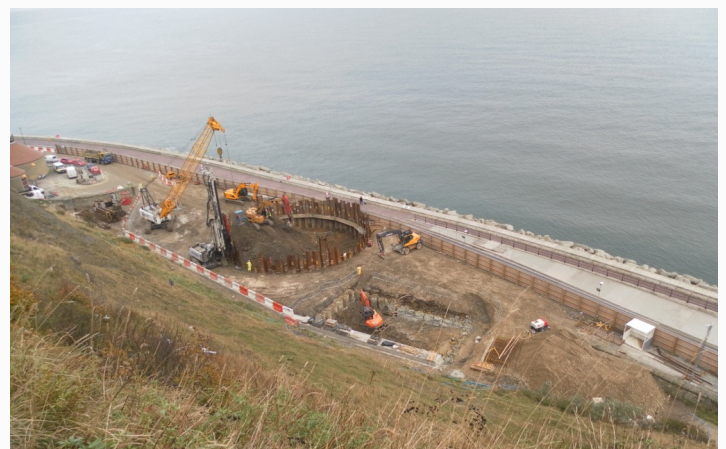
October - work starts on the storm water tank
